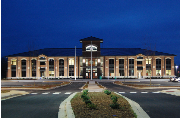
Administration building, Gaffney, South Carolina
